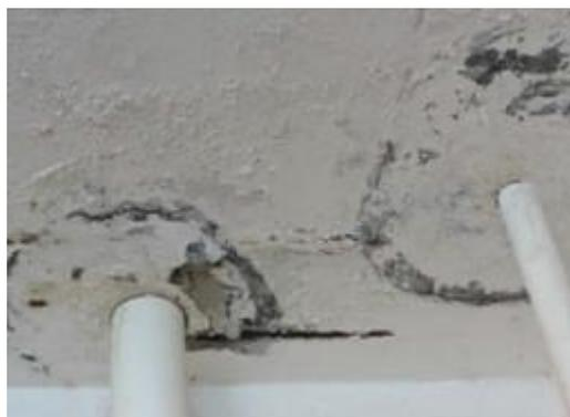
**Figure 11.** Cracking on the edge of planter box and deterioration of waterproofing on slab surface
