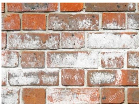
Figure 3. Salt crystallisation on brick wall
