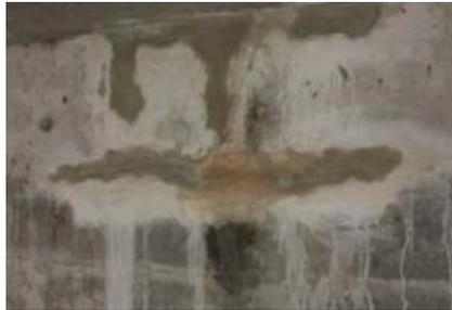
**Figure 10.** Leaking that can be found on the swimming pool wall
