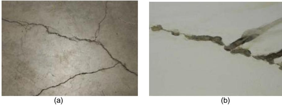
**Figure 5.** (a) Cracking on the floor (b) spalled concrete
