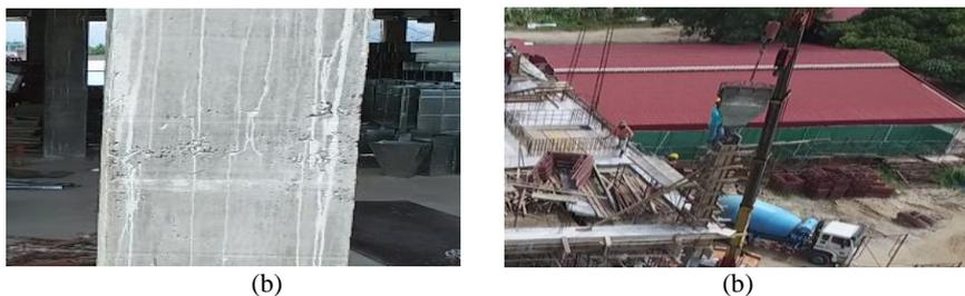
**Figure 8.** (a) Honeycomb defects, (b) concrete casting work in progress
