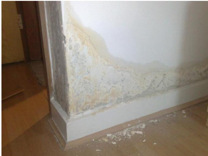
**Figure 5.** Rising damp on masonry wall
