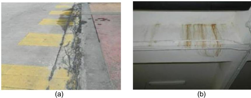
**Figure 7.** (a) Expansion Joint on the Parking lot surface and (b) the effect on structure below
