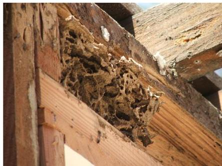
**Figure 2.** Termite damage on building structure
