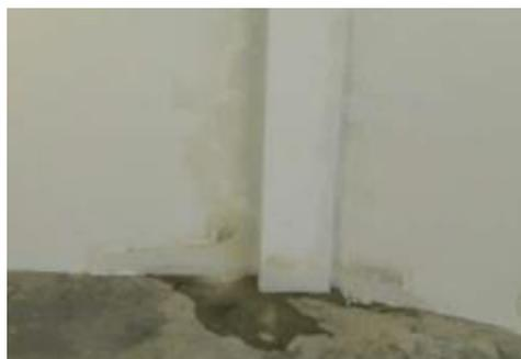
**Figure 0.** Imprint of water caused from rising damp
